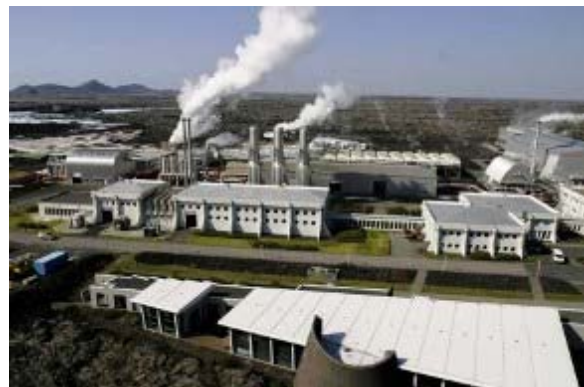
Figure 1. The geothermal power plant of HS Orka in Svartsengi, Iceland.
